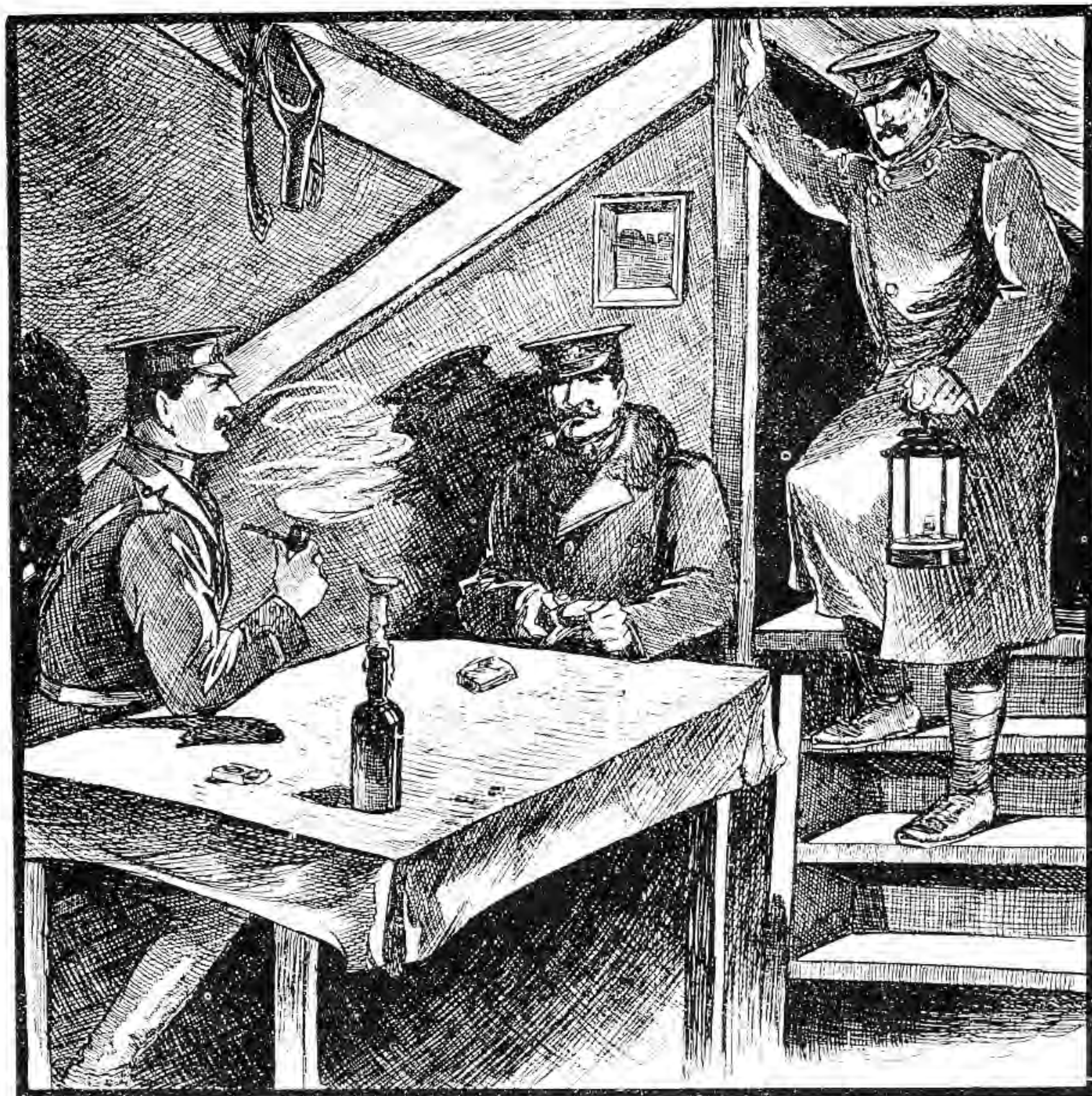
Although one hears a lot about the flooded trenches of Belgium, knee-deep mud and water is not always the case. In certain favourable situations our cheerful Tommies manage to construct for themselves comparatively comfortable quarters, to which they retire when their arduous duties in the trenches entitle them to a spell of well-earned rest, and in the above illustration our artist depicts a typical scene in one of these cosy shelters.
