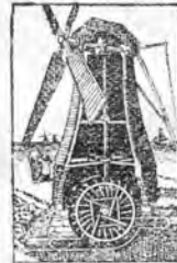
How a Dutch wind-mill pumps out water
